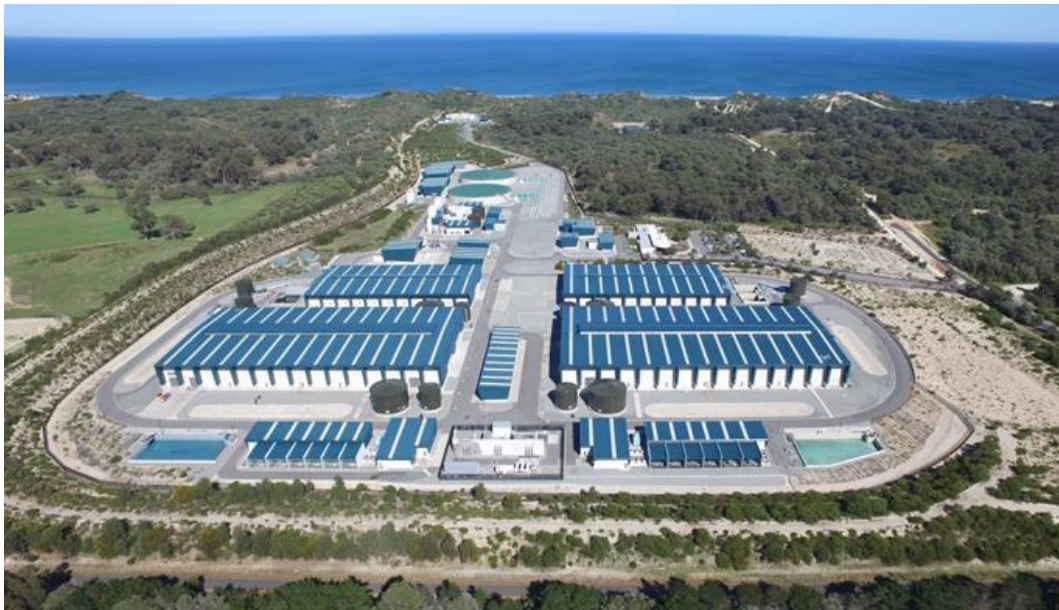
Figure 8: The Southern Seawater Desalination Plant, Perth
