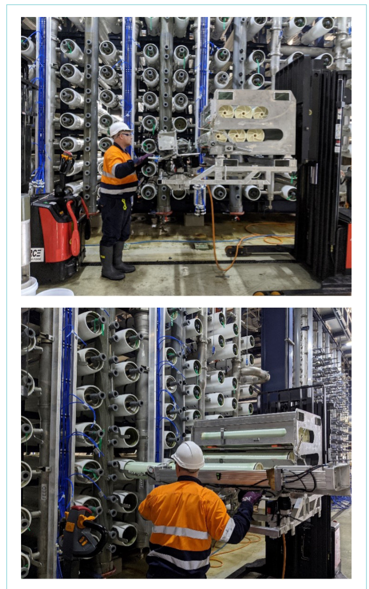
Figure 3: Second Pass BWRO membrane replacement with the semi-automated membrane loader
