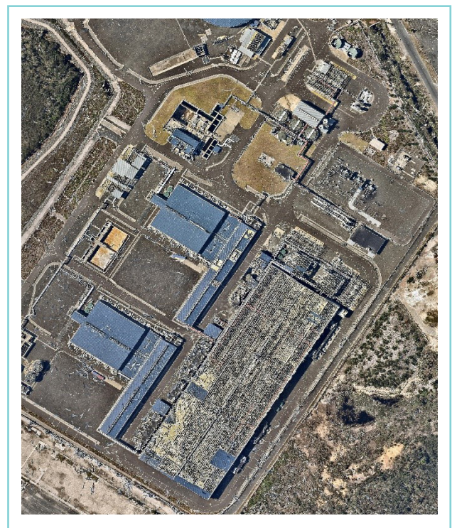
Photo 2: SDP immediately after the storm
