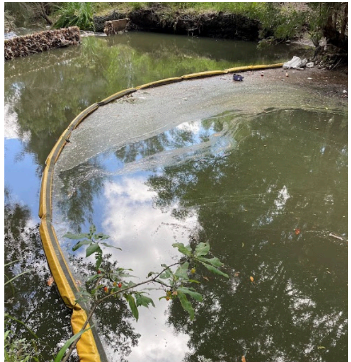
Figure 2: Silt curtain being trialled at Botany Wetlands Canal, Sydney
